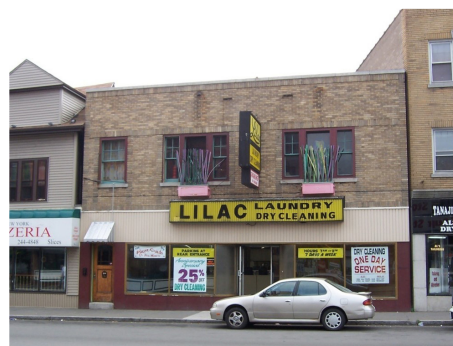
Removing, covering, or significantly altering facade details and/or openings.
