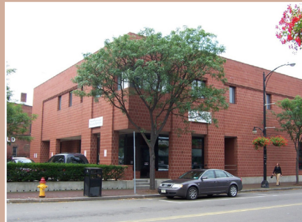
Limited variation in building material and blank facades.
