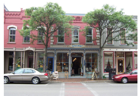
Maintenance, repair, or replacement in-kind of architectural detailing.
